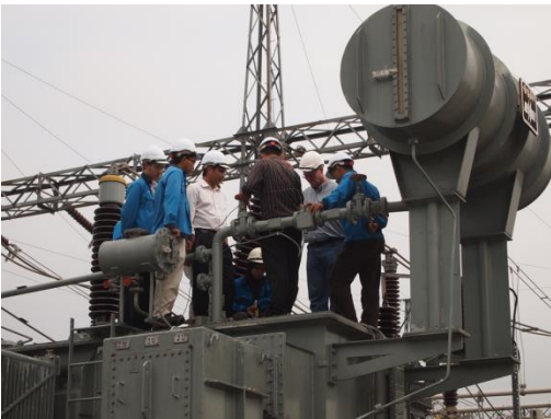
4.) Opening the OLTC head cover to remove the diverter switch
